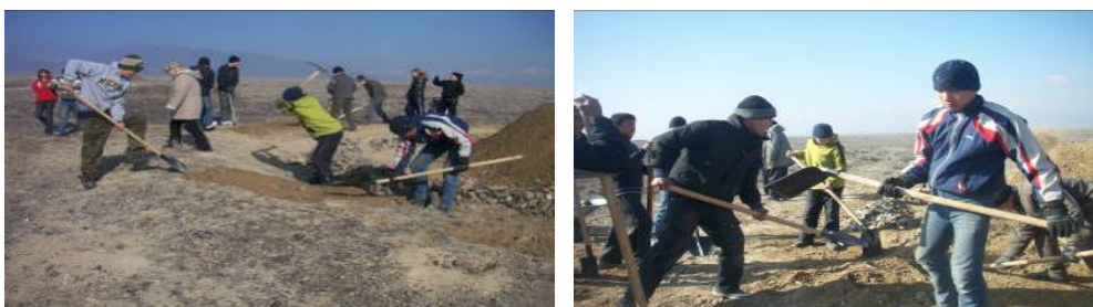
Figure 5 - The work is in full swing
